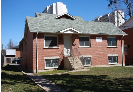
Image 1: Street view of the front of 310 King, Unit 1 entrance.
