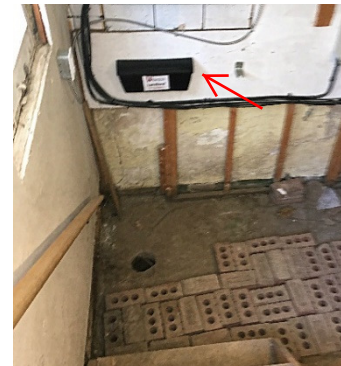
Image 5: Stairwell leading into lower basement laundry room.
