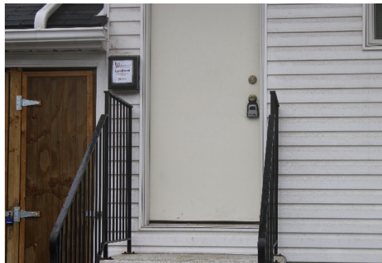
Image 2: Rear door at the back of building with the landlord's mailbox.
